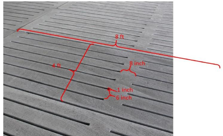
**Figure 2: Photographic view of a portion of the barn floor.**
